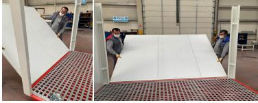
3)THE PANELS ARE PLACED INTO THE SOCKETS ON THE SUMP BY THE PINS IN THE SUB-SECTIONS OF THE PANELS.
