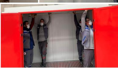
7)THE ROOF IS PLACED AS SHOWN IN THE IMAGE AND IT IS READY TO BE CONNECTED TO LIFTING BRACKETS
